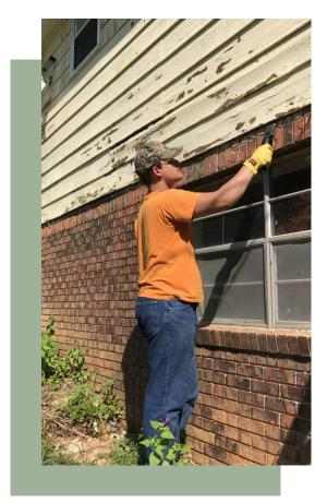
DISTURBING LEAD-BASED PAINT WITHOUT CONTAINMENT H&S §17960 | THE BUILDING
