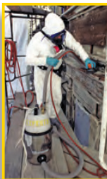
Attach power tools to a HEPA vacuum.
